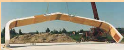
Newood, industrial building, length 30 m, free span 15 m, height 6 m, shell thickness 0,40 m, with a canopy and sliding Newood doors.
