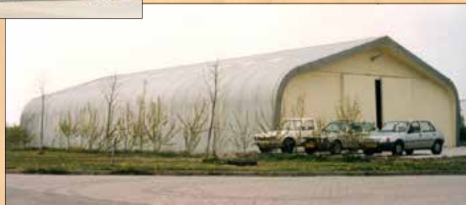
Newood, industrial building, length 30 m, free span 15 m, height 6 m, shell thickness 0,40 m, with a canopy and sliding Newood doors.
