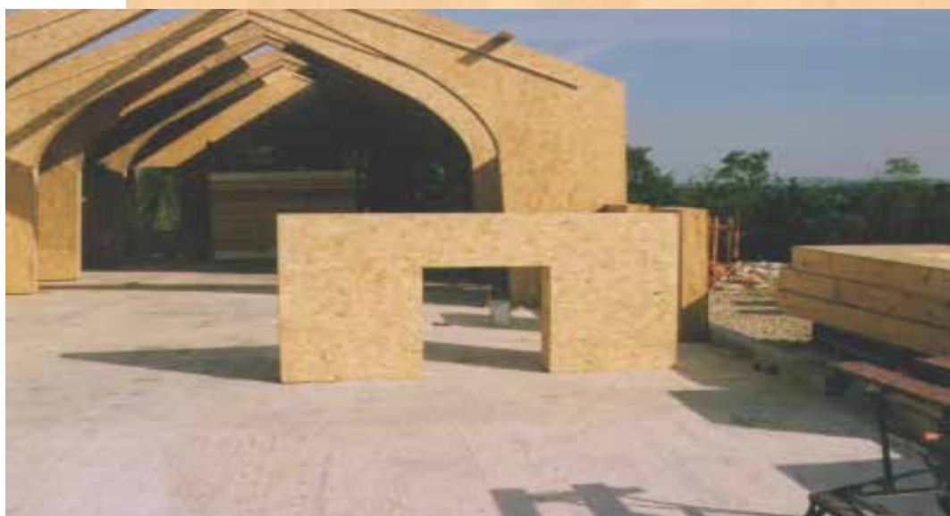
Newood/Jasse, assembly of two half-arches.
