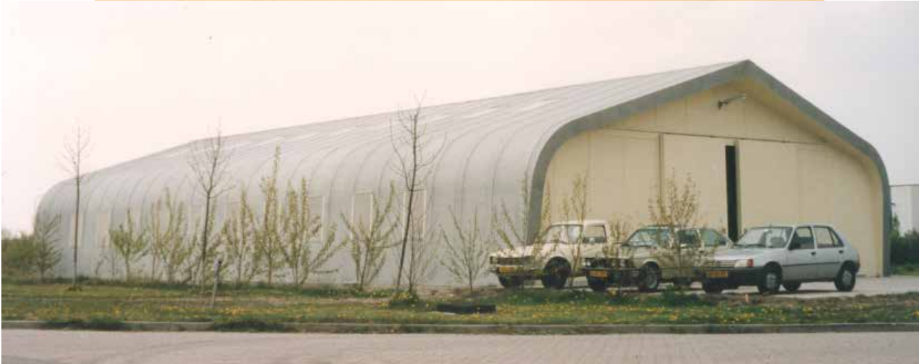
Newood, industrial building, length 30 m, free span 15 m, height 6 m, shell thickness 0,40 m, with a canopy and sliding Newood doors.
