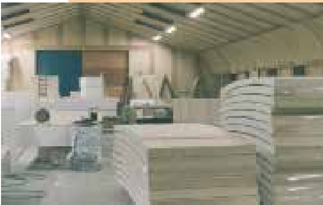
Newood, industrial building, length 30 m, free span 15 m, height 6 m, shell thickness 0,40 m, with a canopy and sliding Newood doors.
