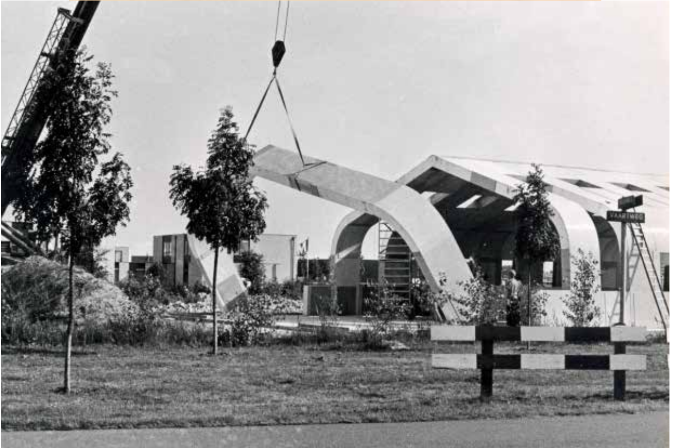
Newwood industrial building, end of the shell segments assembly.
