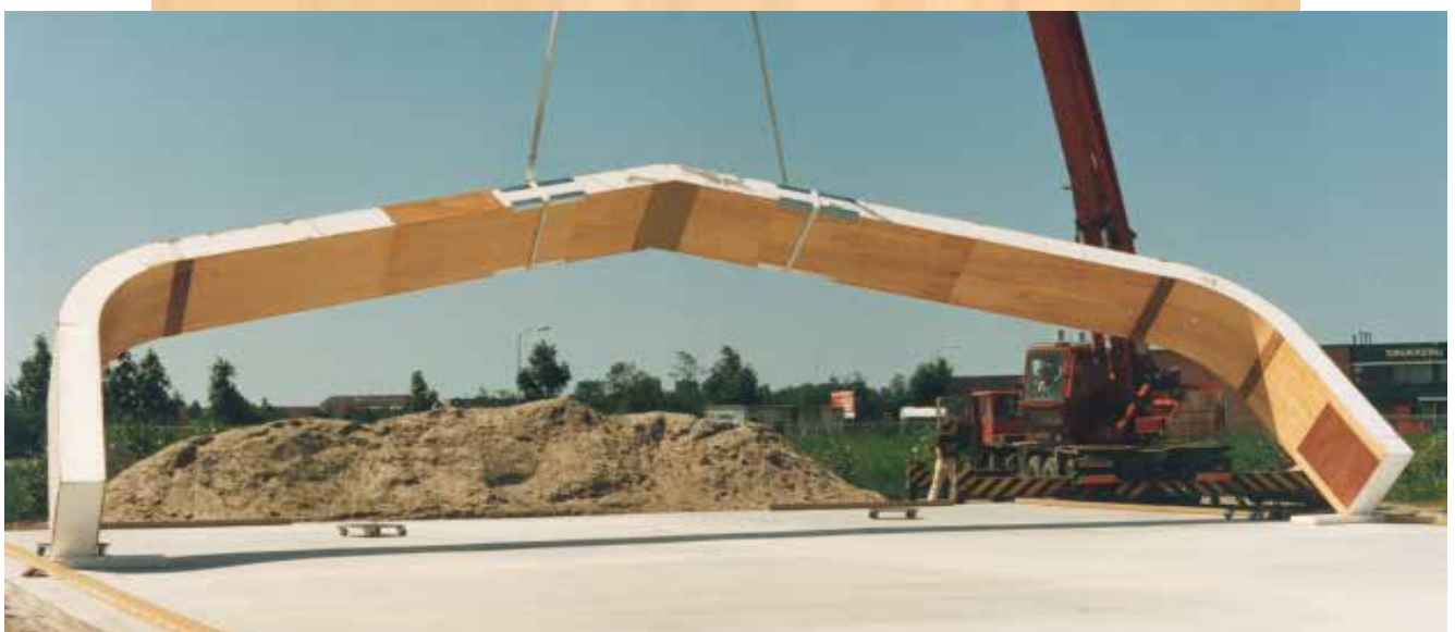
Newood, industrial building, shell segment 1,25 m large by a thickness of 400 mm. Free span is 15 meters.
