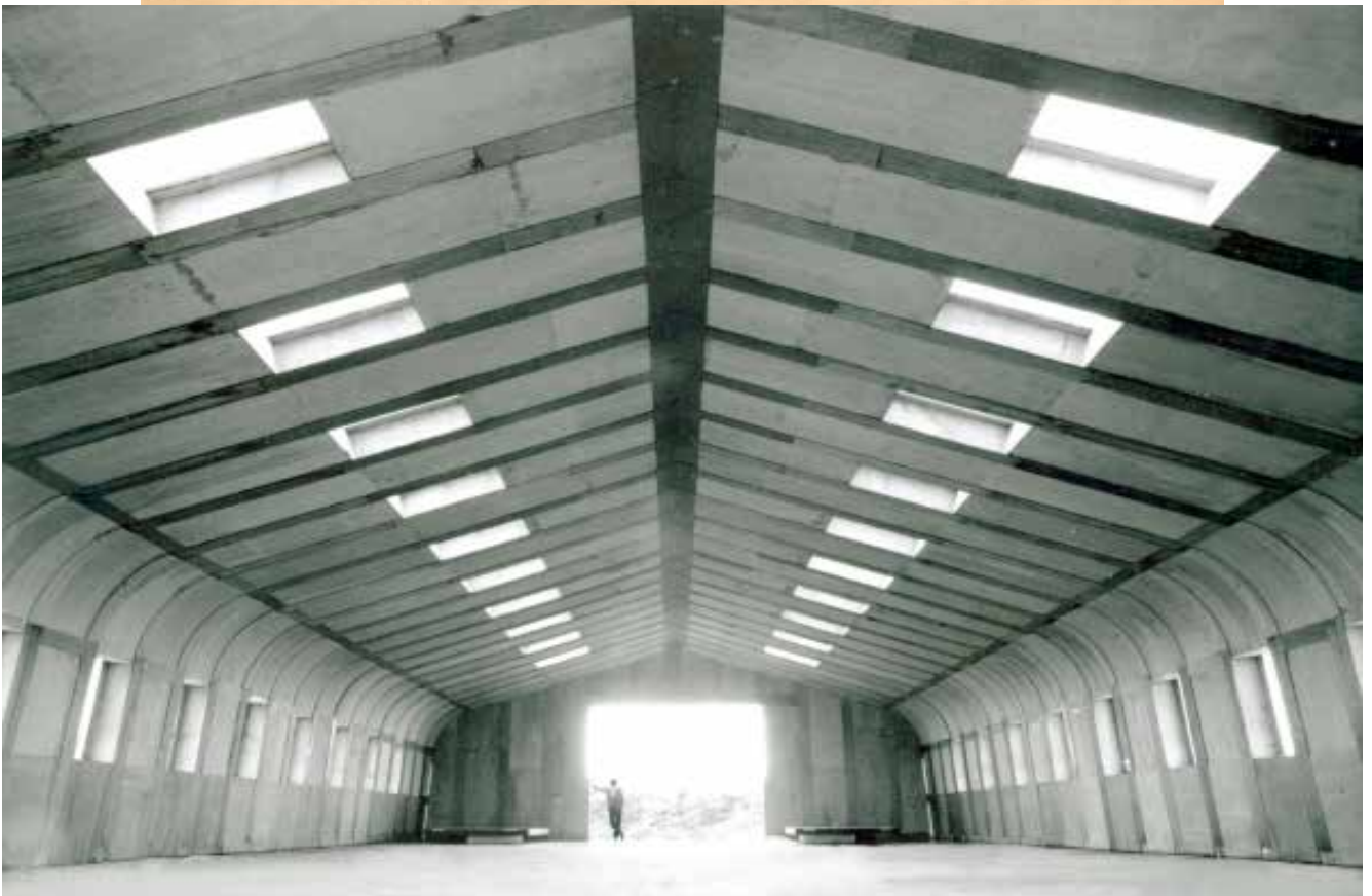
Newwood, industrial building, the inside building shape.
