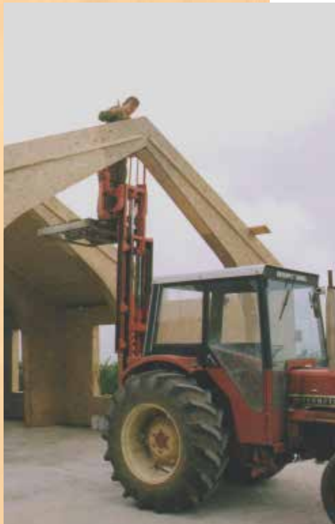
Newood/Jasse, assembly of two half-arches.
